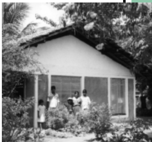
Oversize bricks; new houses for many
